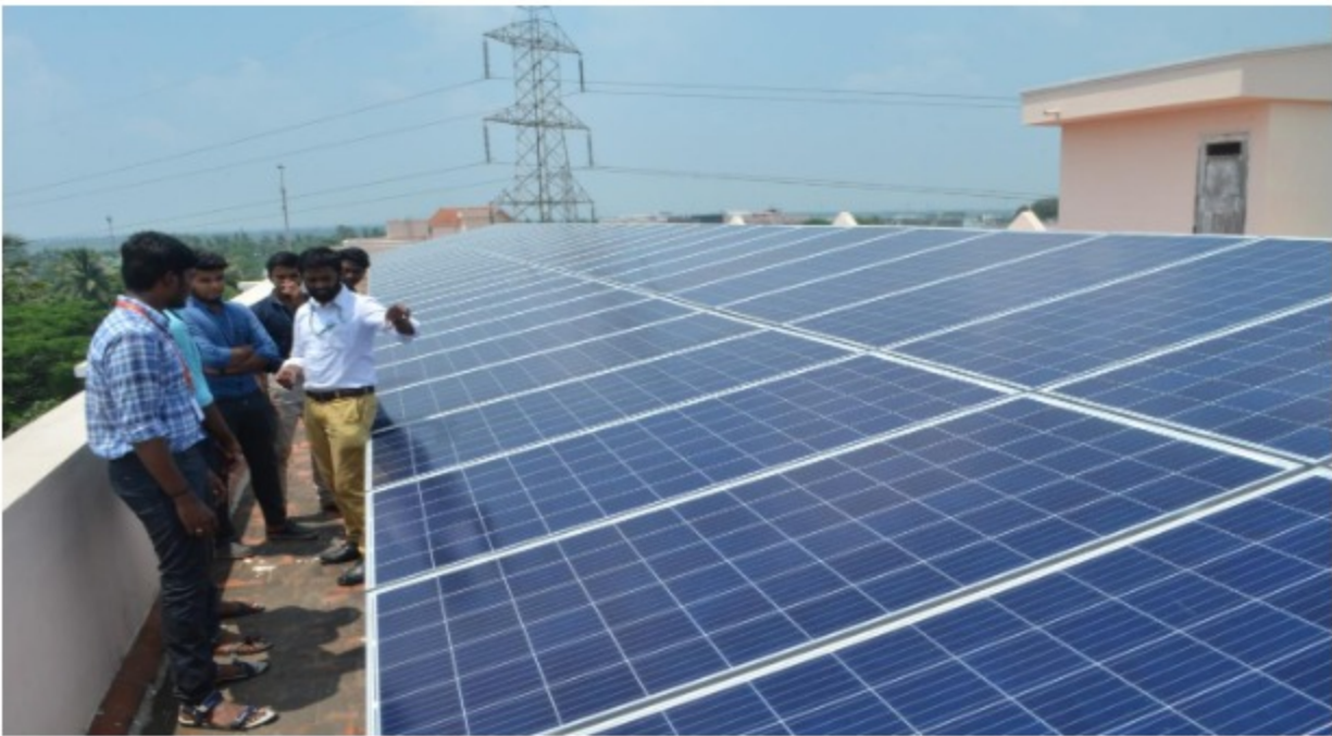
20KW Roof Top Solar Power Grid
